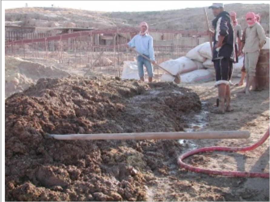
Illustration 55: Mud mixture for mudbrick production; note AP Palace in background (MZ V22i2235).
