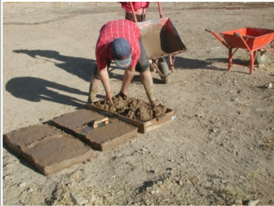
Illustration 58: Pressing mud-mixture into the form (MZ V22i2236).
