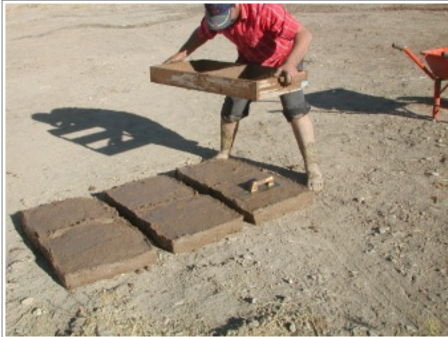
Illustration 59: Removing the brick form (MZ V22i2162).
