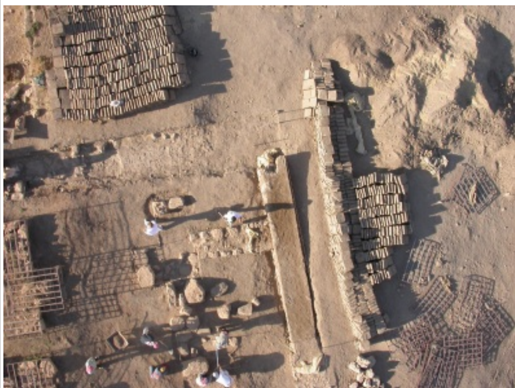
Illustration 94: Overhead photo of the reconstruction project at the AP Palace. Note the mudbricks stacked in the top and right of the image, soil for plaster in the upper right, as well as the stones in the lower right (MZ V22i2240).
