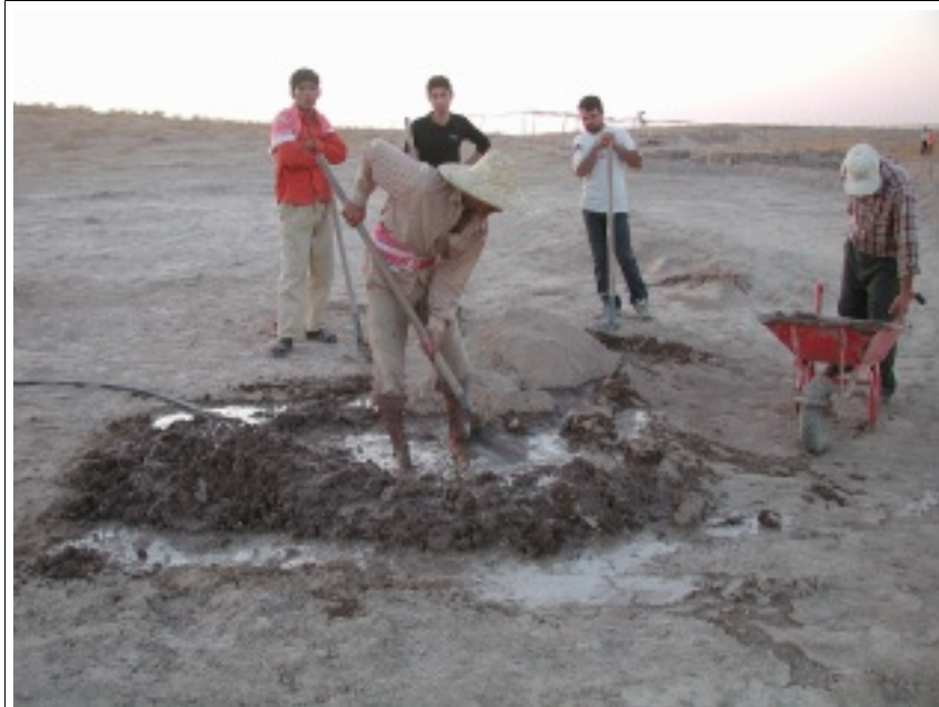
Illustration 70: Mixing dirt and water for plaster.
