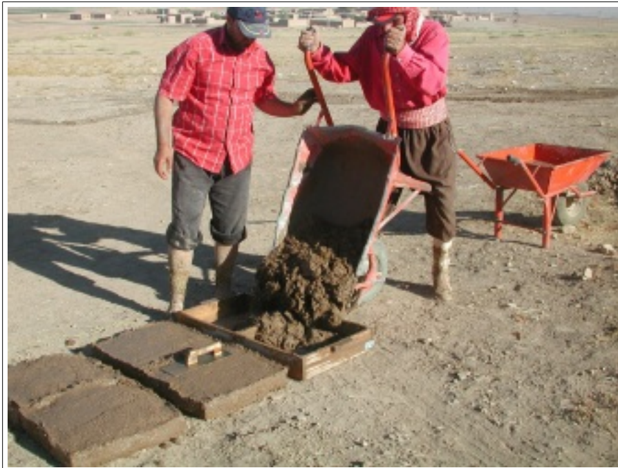
Illustration 56: Adding the mud-mixture to the brick form (MZ V22i2159).
