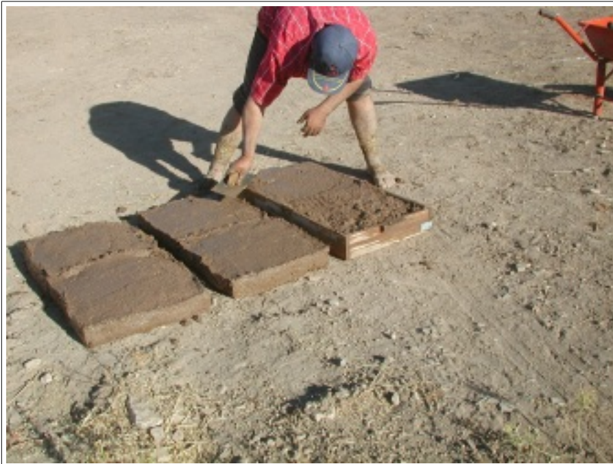
Illustration 57: A trowel is used on the top (MZ V22i2161).
