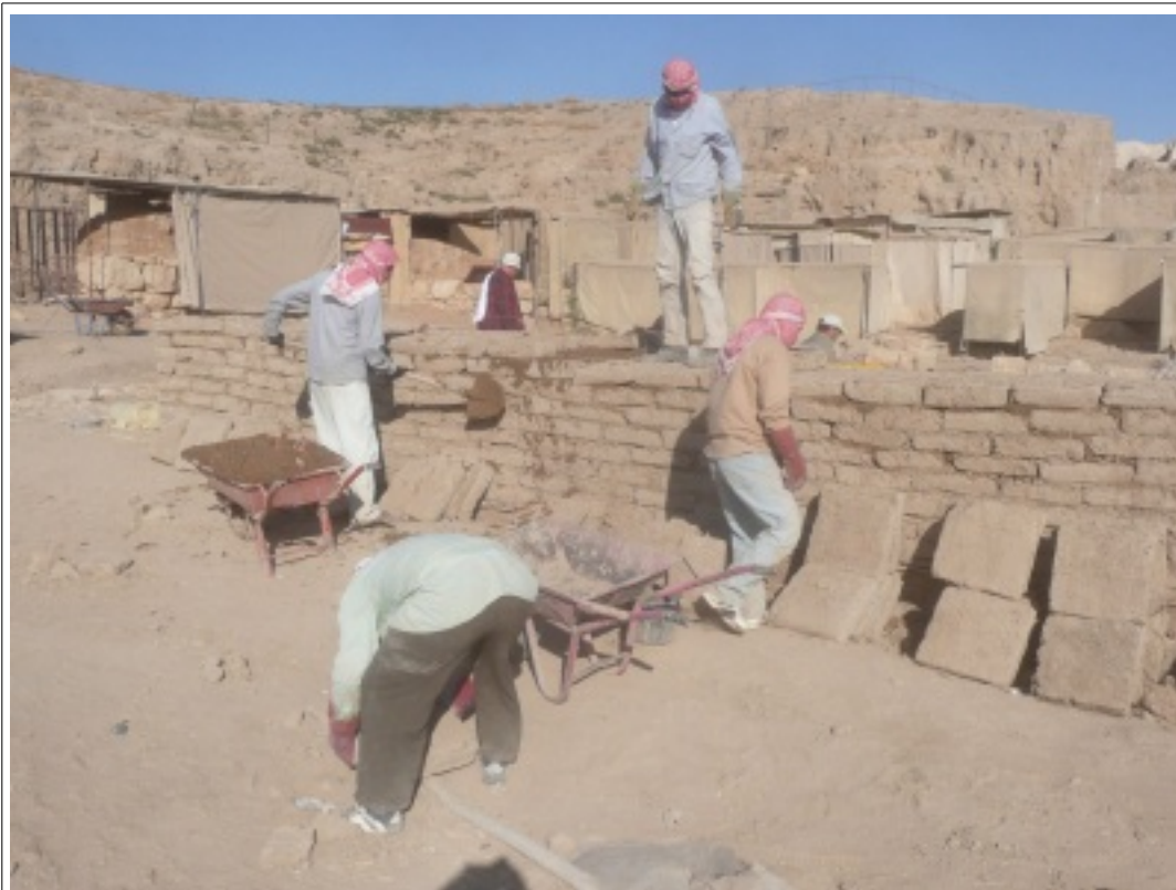
Illustration 100: Wall construction during the reconstruction of the destroyed walls of the AP Palace. Note the workman 'splitting' a brick into two half-bricks over a pole in the foreground (MZ V22i2241).
